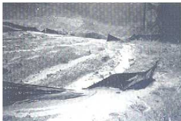
High clay turbidity in runoff water from bare soil at a construction site.
